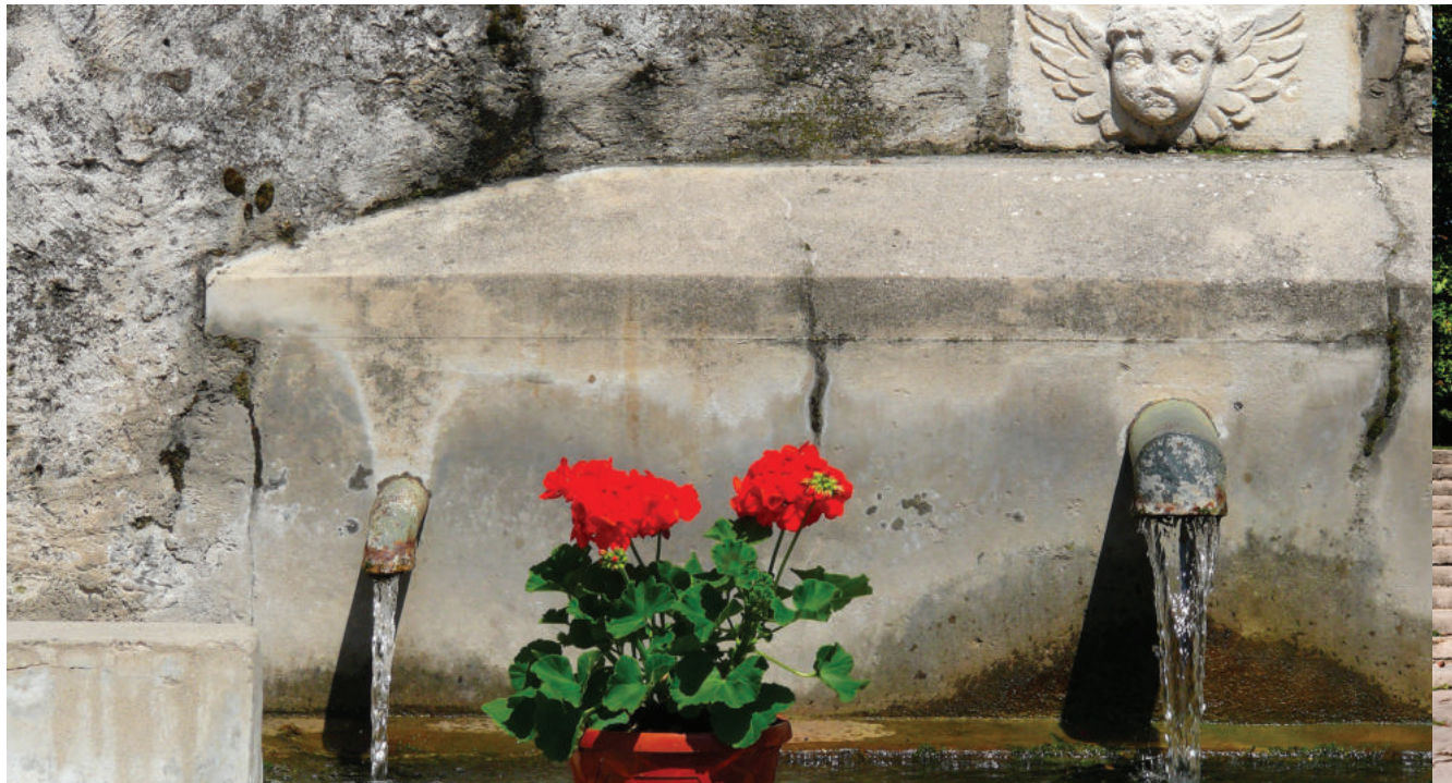
Lavatoio, via Roma Wash house, via Roma
